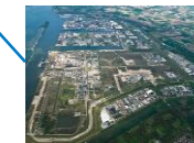
Port of Moerdijk
